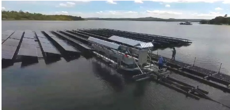
The picture shows the solar power plant project installed on the water at Sirindhorn Dam, size 256 kilowatts.
