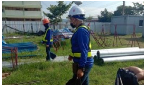
5S activities in work area
